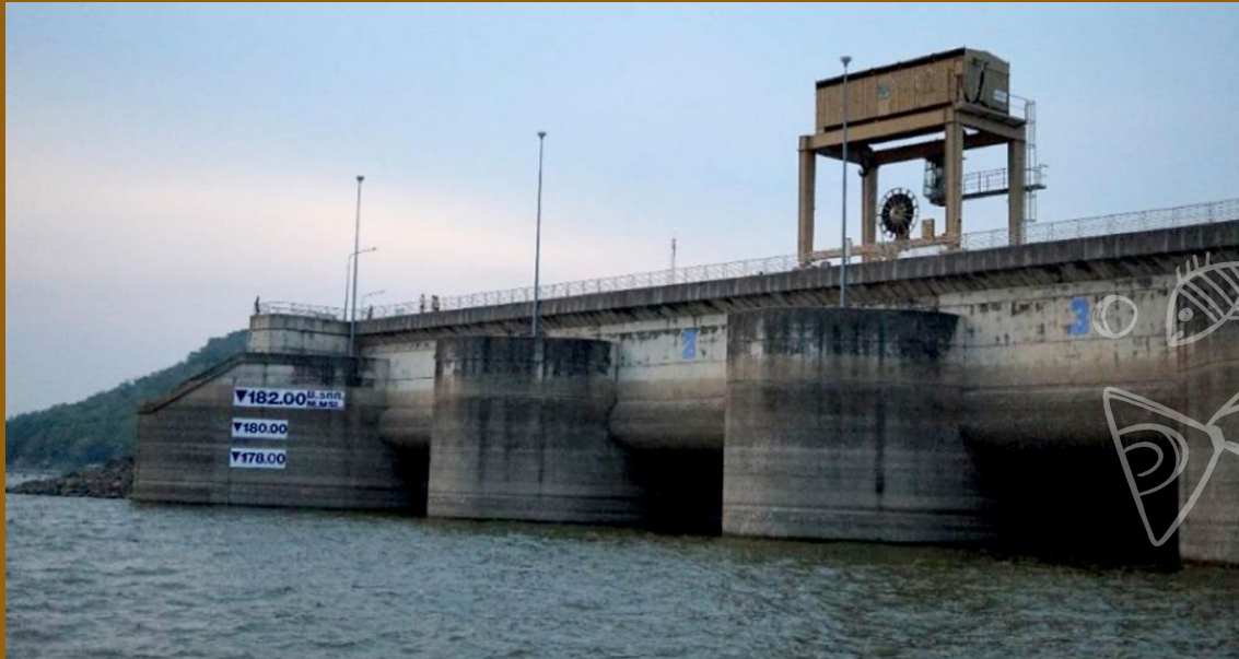
Ubolratana Dam Reservoir
