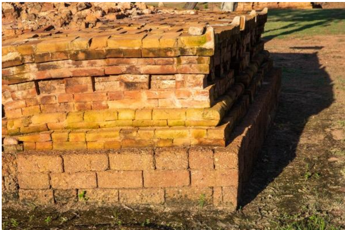
SiThep160 The Luad Bua brick laying method applied at the base of subordinating pagodas
