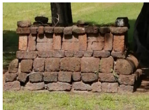
Figure I-3-14 The base of the stone Dharmachakra made of laterite brick laid to form small rooms
