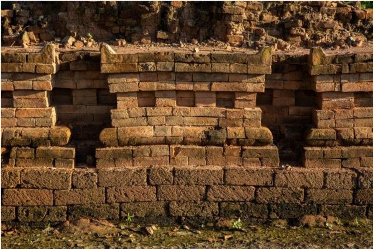
SiThep160 The Luad Bua brick laying method applied at the base of subordinating pagodas
