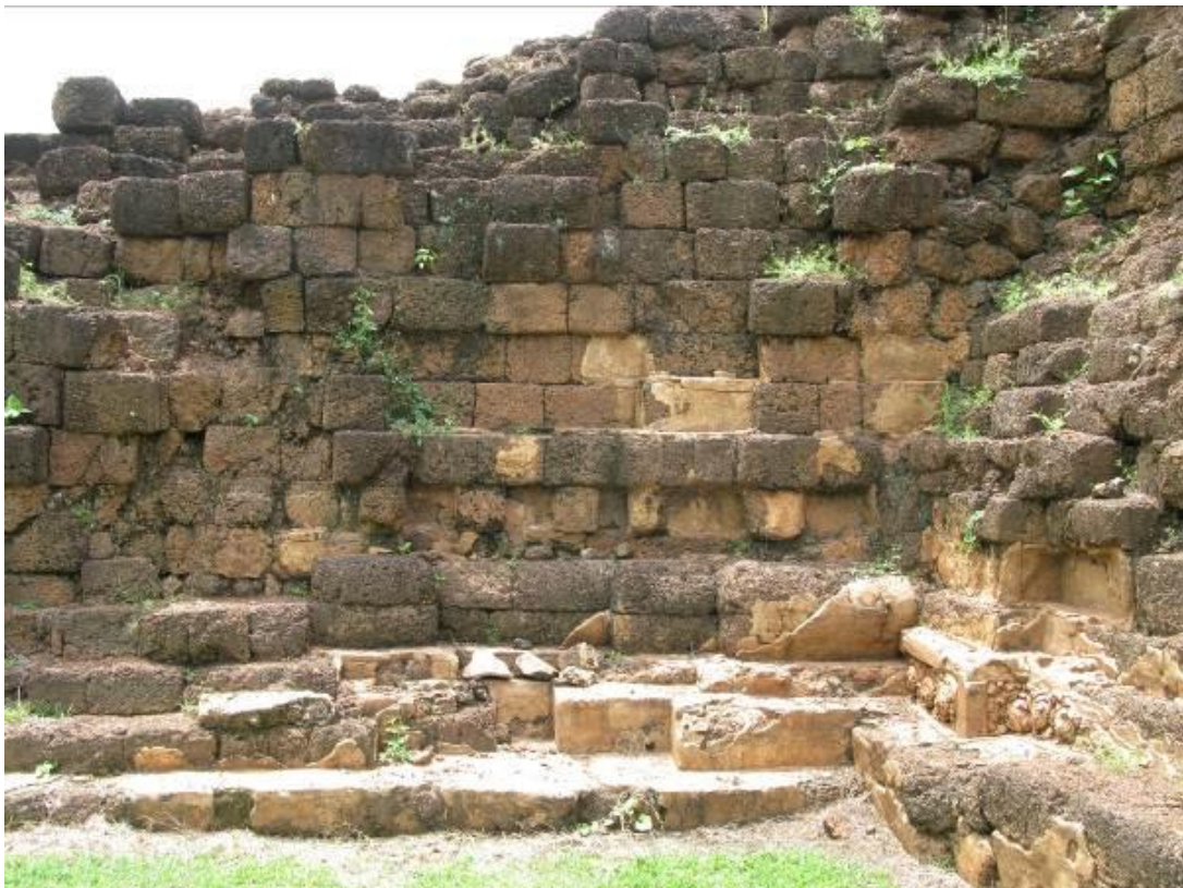
Figure 2-19 The Bua Valai base and the indented corners system, Khao Klang Nai, Muang Si Thep, Phetchabun Province
