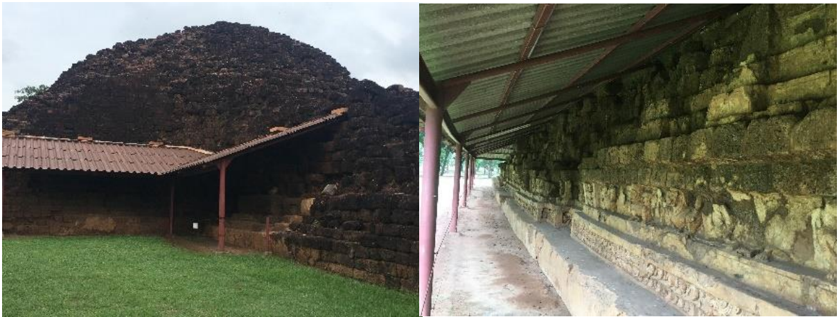
Figure 4-8 The roof tiles for protecting the stuccos, Khao Klang Nai
