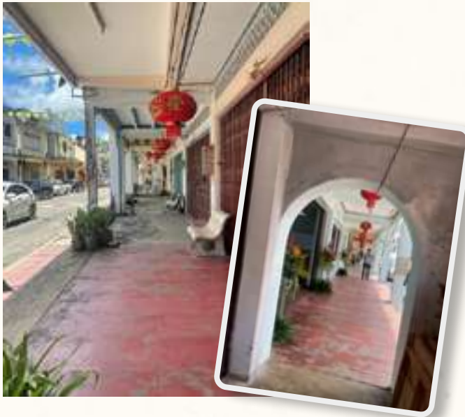
Ngo Ka Khee or the shared arcade walkway beneath the buildings
